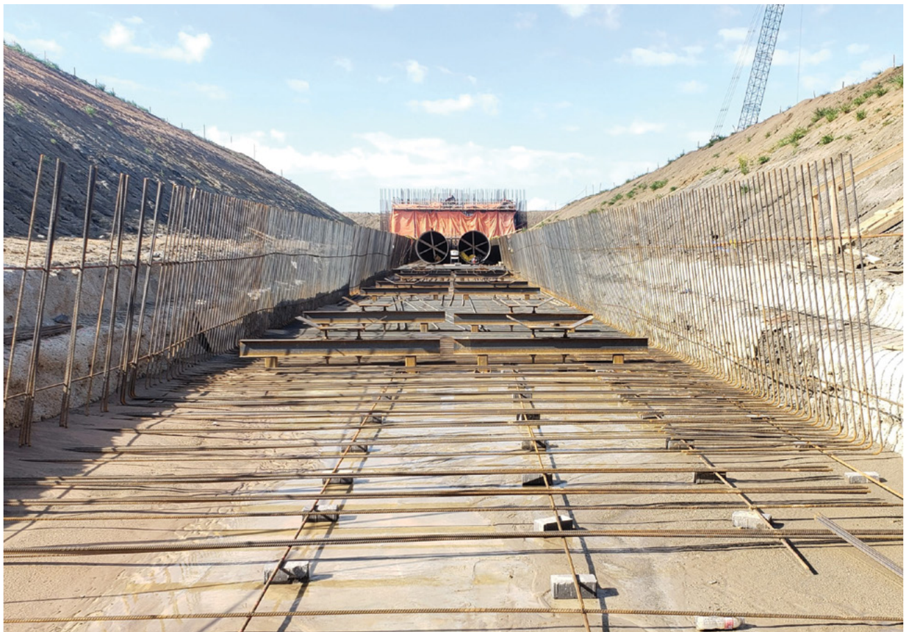
Intake structure at Bois d'Arc Lake; photo courtesy of North Texas Municipal Water District
